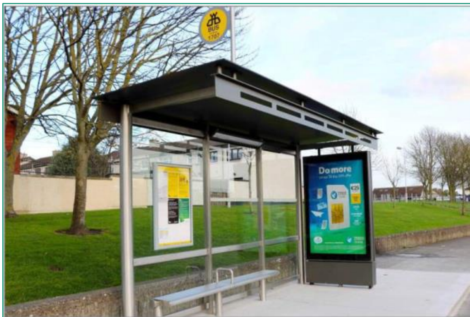
Figure 2.3.5.22: Standard 3 Bay Reliance Mark Shelter with full width advertising panel
