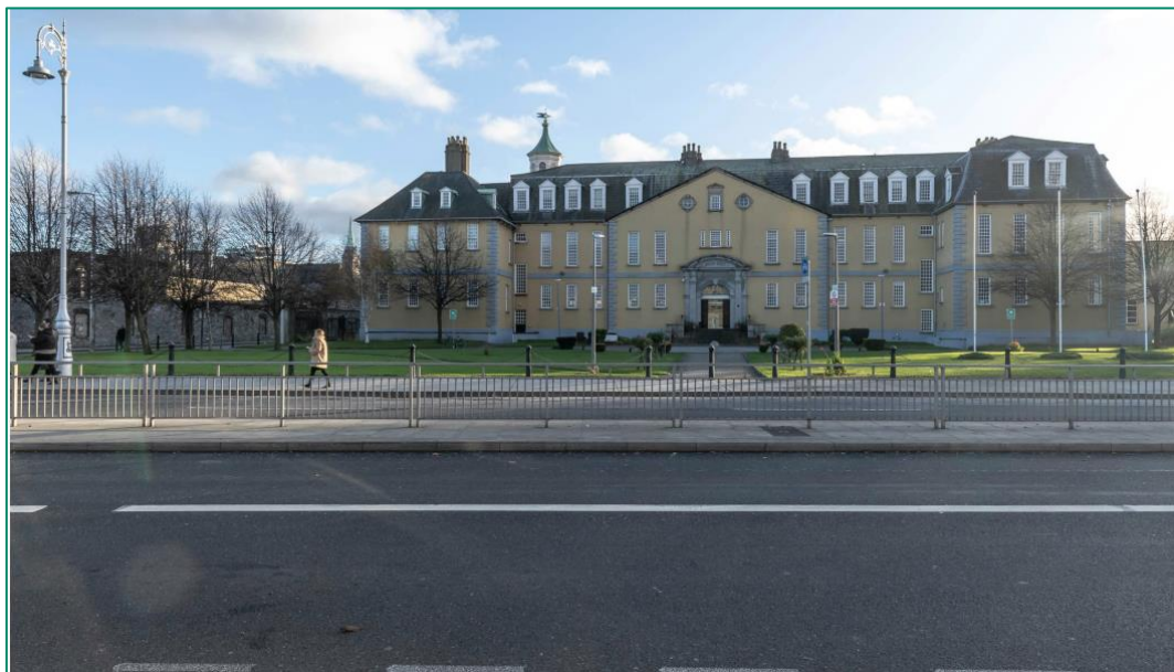
Figure 2.3.5.20 View 07: As existing view of Dr Steevens' Hospital
